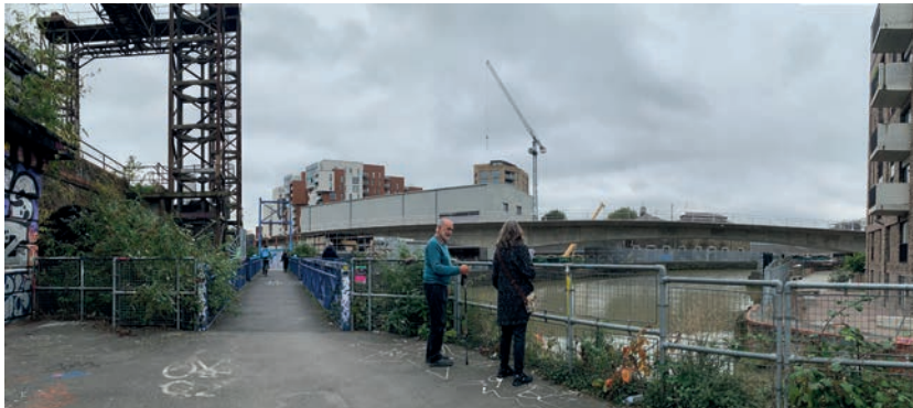
View towards DLR bridge and Thames Water site
